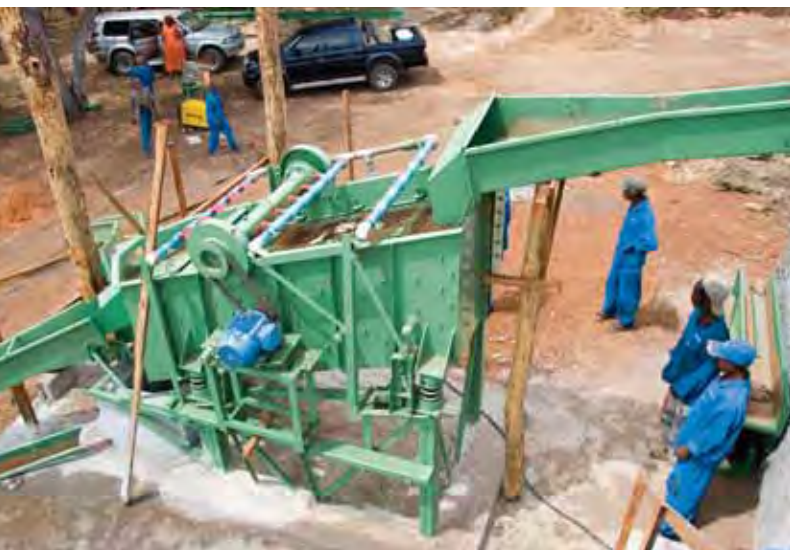
Figure 32. Future mining for Cu-bearing tourmaline by Mozambique Gems will employ this washing plant. Photo by B. M. Laurs.
