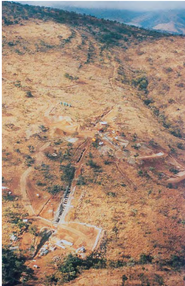
Figure 1. This aerial view (looking east) of part of the Klipsinger project shows the Leopard "fissure." The dike is about 1 m wide, and is visible over a distance of approximately 1 km in this photo; drilling has shown it to be 3 km long. The first underground adit at this fissure is visible in the foreground. Photo courtesy of SouthernEra.
