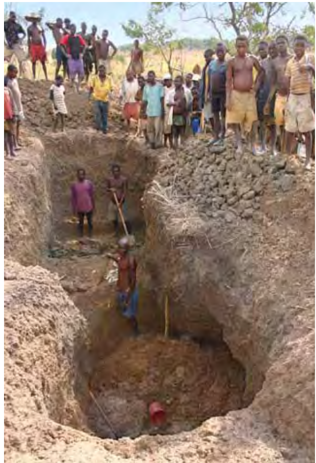
Figure 28. Miners work the Muva tourmaline deposit with picks and shovels in a series of shallow pits. Photo by J. C. Zwaan.
