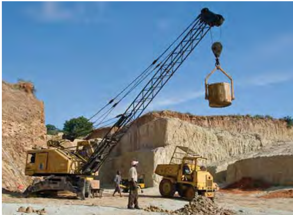
Figure 16. Cranes are used to remove the excavated material from the shafts, as shown here at the Kimbo pit. A cage that is used for hoisting the miners is visible in the dump truck. Photo by B. M. Laurs.
